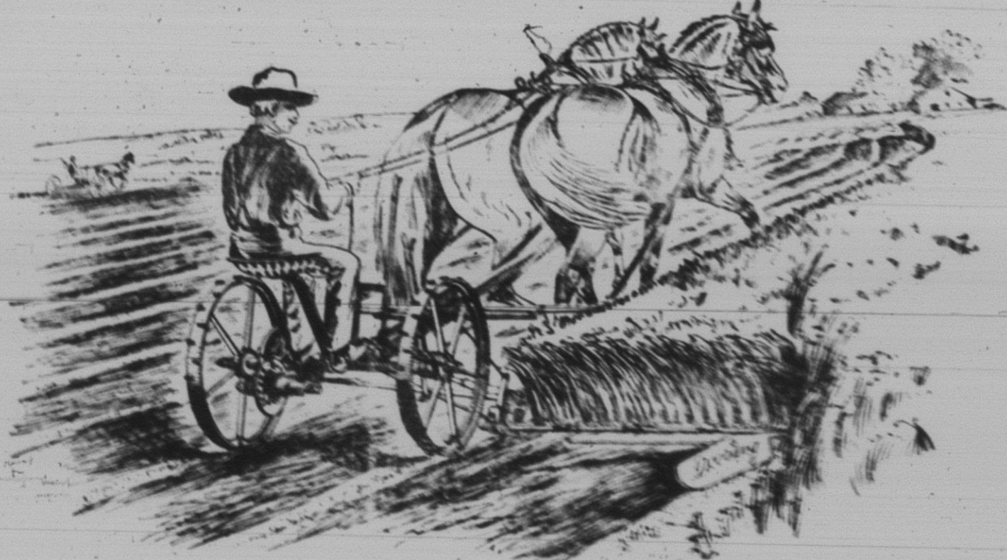
Deering Ideal Mower, Roller and Ball Bearings.
